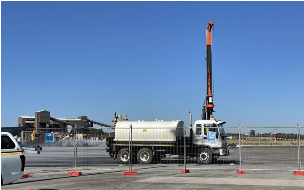
Figure 9: Environmental Inspection Showing Water Cart in Use
