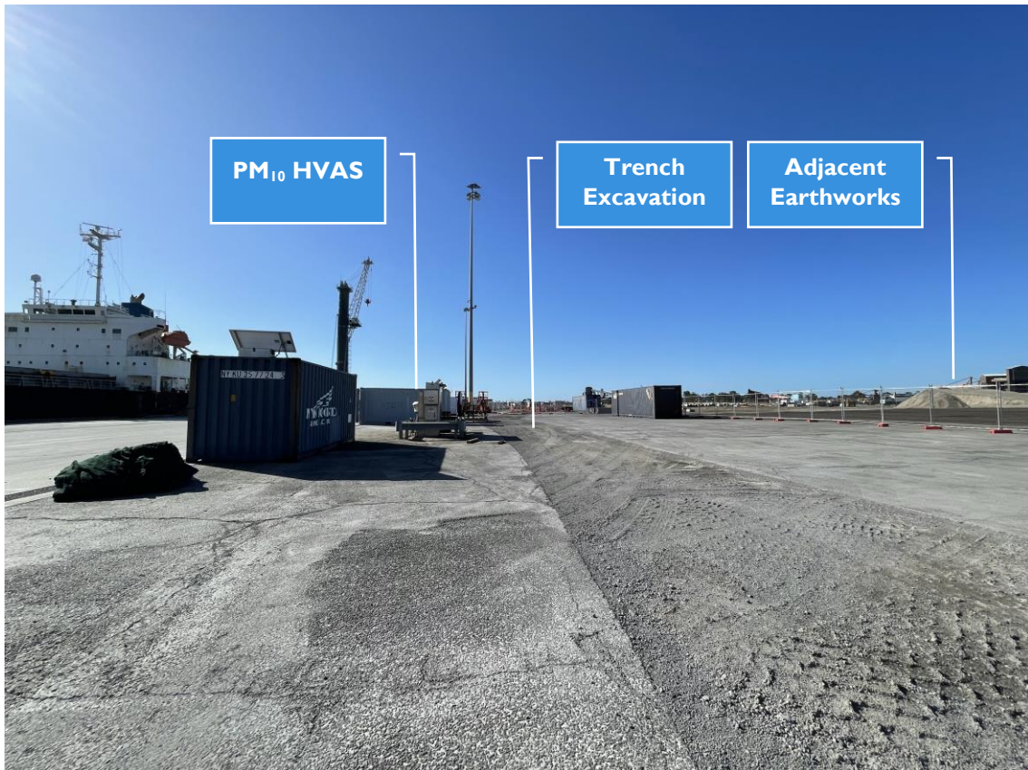
Photograph 2: Trench Excavation in Close Proximity to PM 10 HVAS
