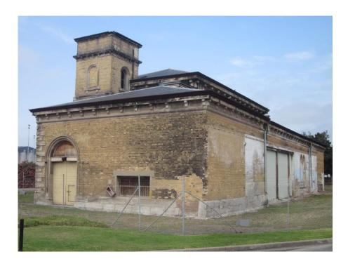
Caption: Eastern elevation; former chimney aperture was originally arched. Pigeons enter through broken tower window.
