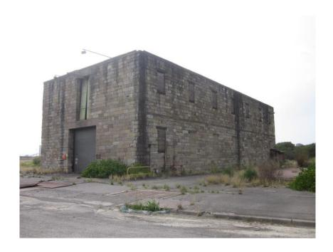
**Caption:** Former BHP Pattern Store, from the south-west; note stone construction and flat concrete roof.
