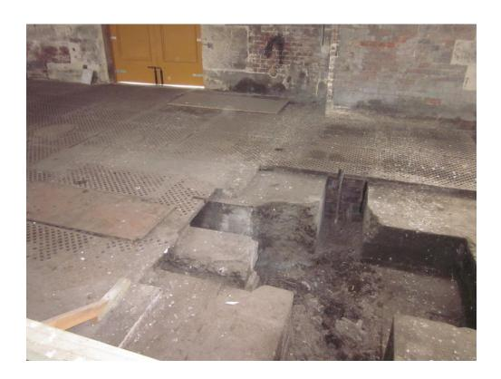
Caption: Void from removed engine, showing iron or steel flooring.
