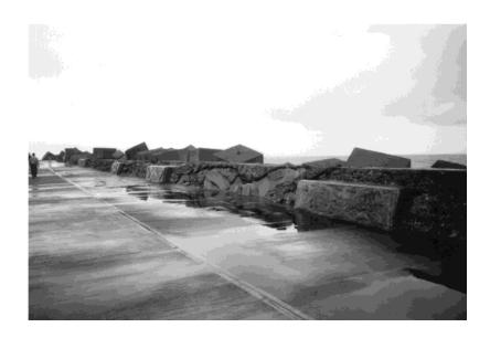
Caption: Detail of the eastern end of southern breakwater, showing mass concrete block wall
