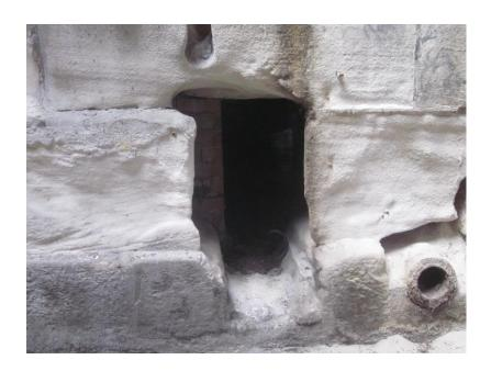
**Caption:** Interior view of the powerhouse, showing deterioration of sandstone.
