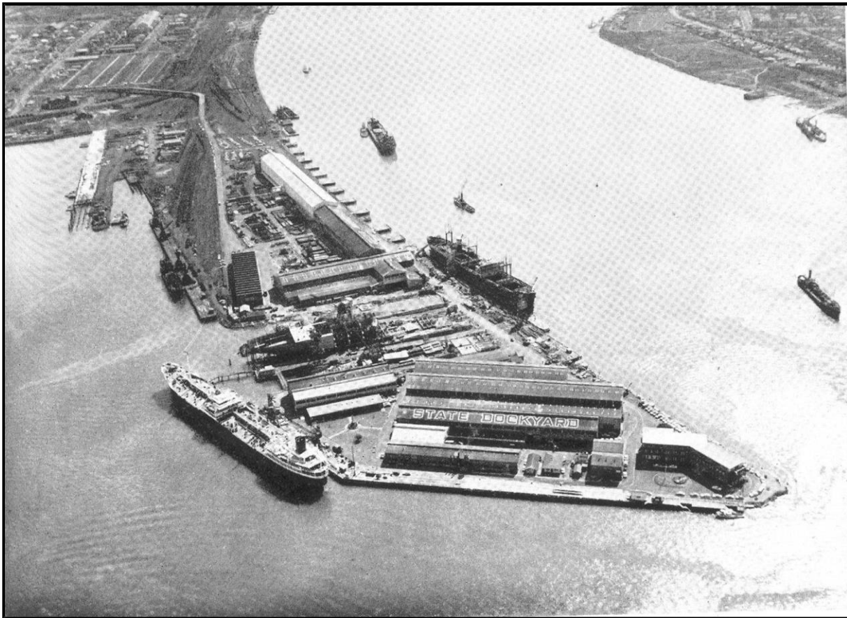
Plate 17: Aerial view of State Dockyard September 1945 The State Dockyard Newcastle NSW, 1945
