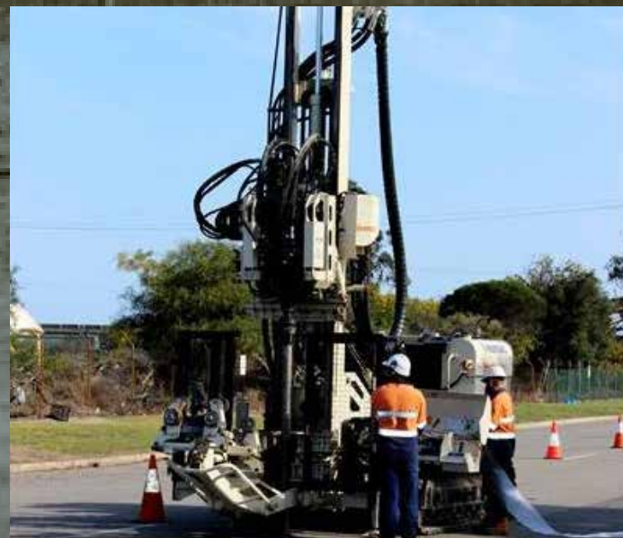
Pictured: a ground water test pit.
